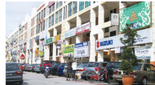
Fortune Square @ Kepong, KL
